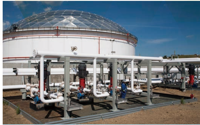
Husky Midstream holds a portfolio of oil pipeline assets in Canada.
