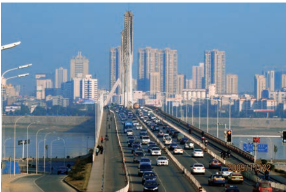
In Mainland China, CKI has a portfolio of investments in toll roads and bridges.
