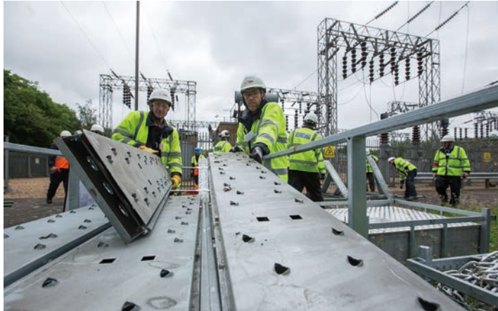
UK Power Networks supplies electricity to London.
