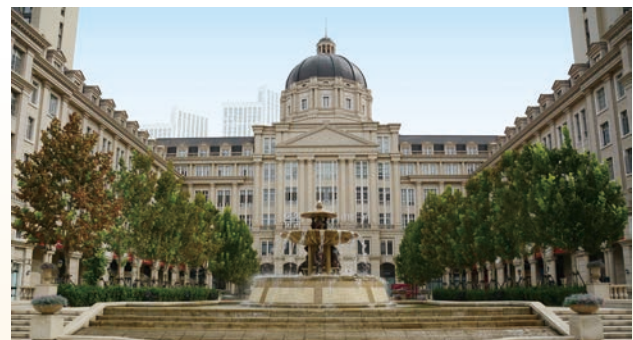
City Plaza (Tianjin)
